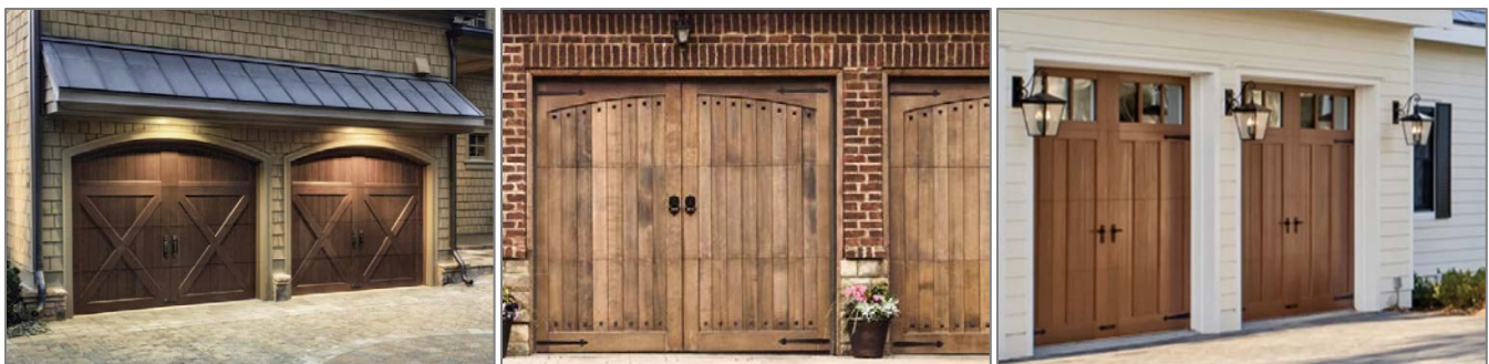
IMAGES 3, 4 & 5: EXAMPLES OF UPGRADED GARAGES
