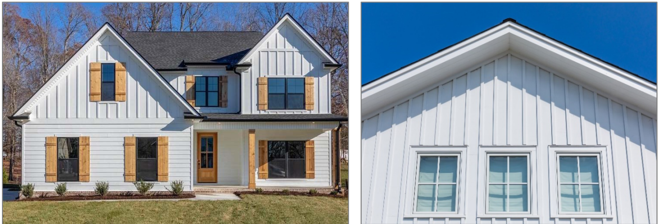
IMAGES 1 & 2: EXAMPLES OF BOARD AND BATTEN FROM THE PLANNED DEVELOPMENT DISTRICT ORDINANCE
