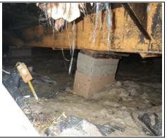
Missing tie down and damaged insulation
